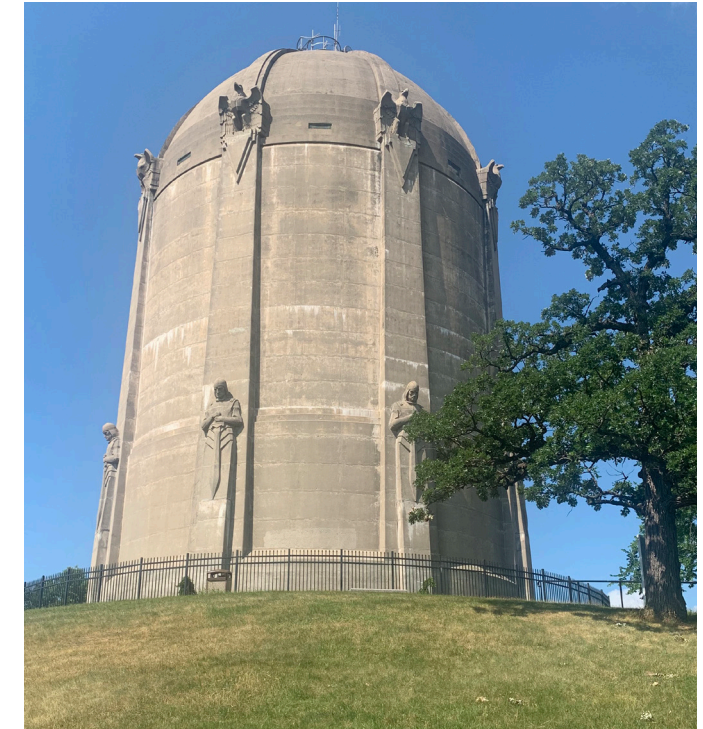
Washburn Park Water Tower.
