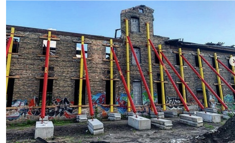
To prevent the walls from caving in, steel supports and joists attached to concrete blocks shore up the building’s exterior. The raw interior still contains abandoned machinery, timber supports, and modern graffiti.
